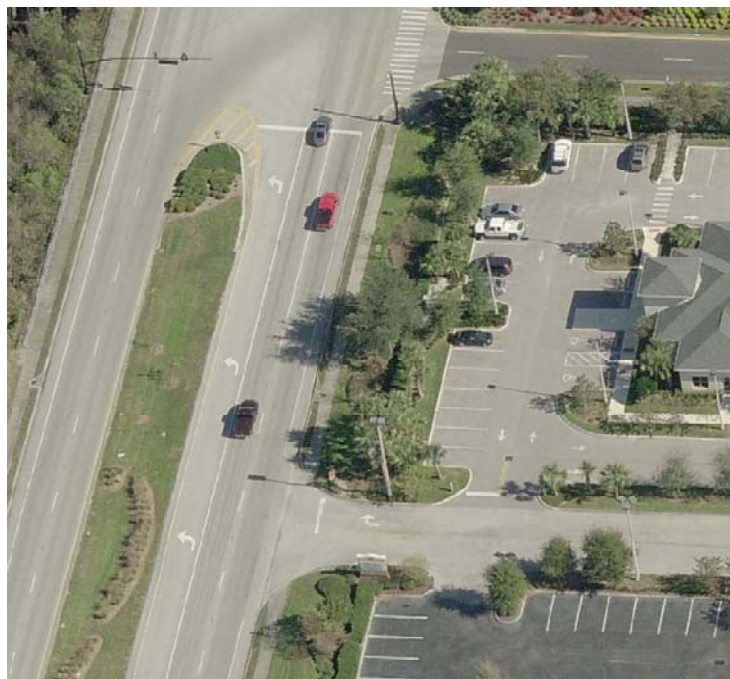
S.R. 434 at Vistawilla Drive – Current Conditions
